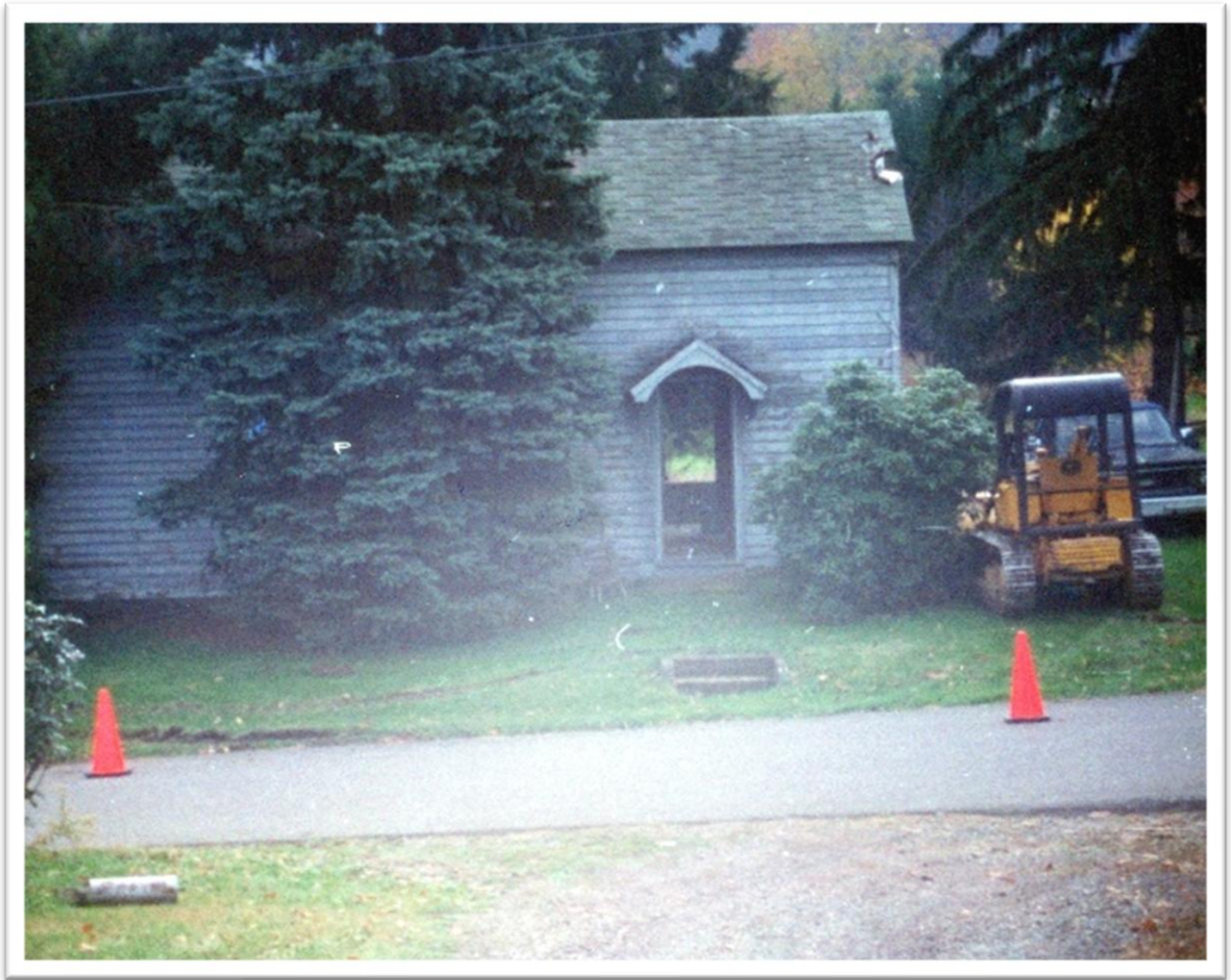
Demolition of Zenith house
