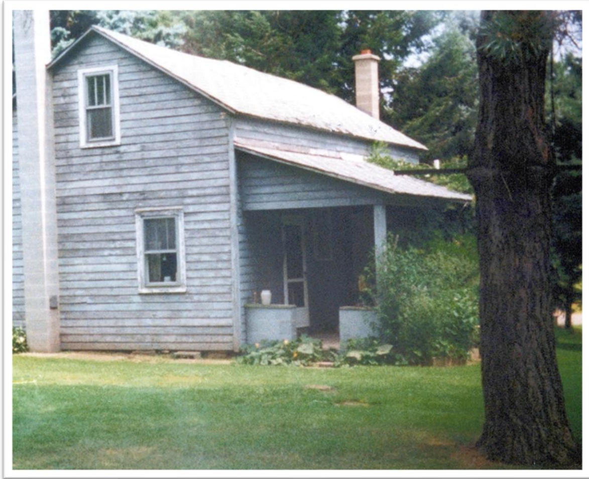
Demolition of Zenith house
