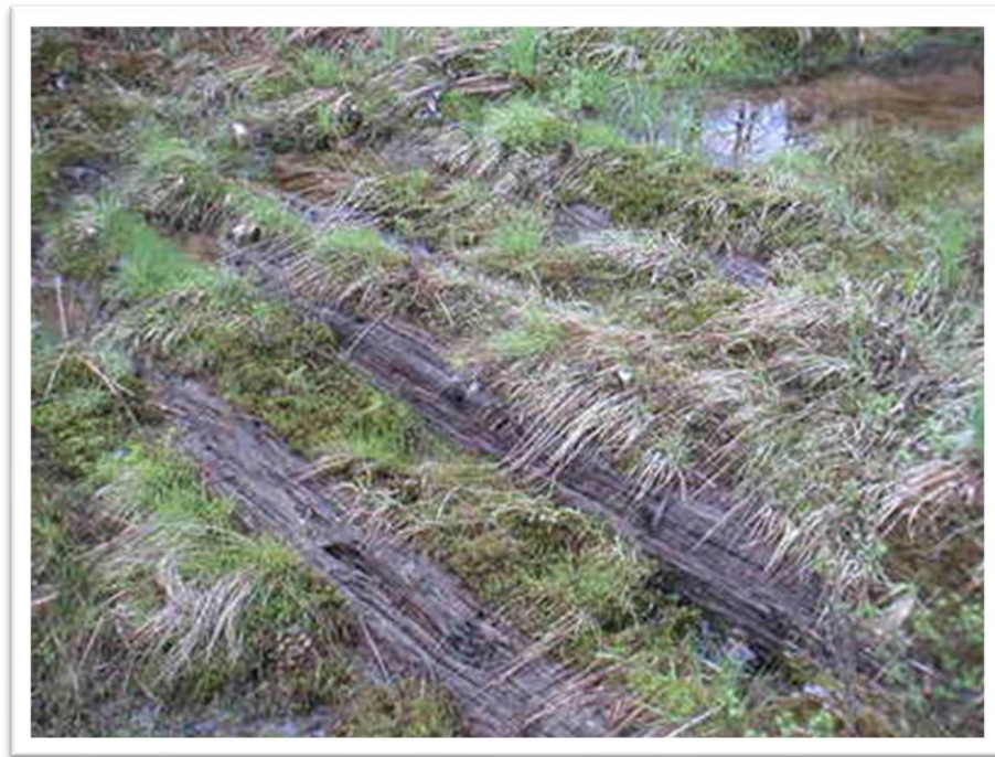
A section of the corduroy turnpike road on Painter Den property, Sullivan County.
